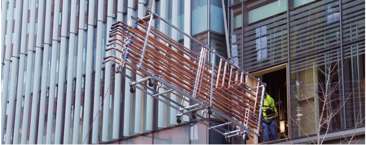
Figure 13. Delivery of a prefabricated utility rack. Source: (Teichloyz, Sarma et al. 2017).
